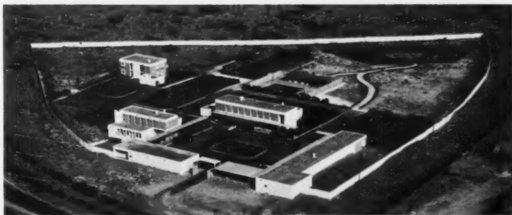
Aerial view of U.S. embassy compound in Nouakchott. White horizontal line in rear is a fence. (Office of Foreign Buildings photo)
